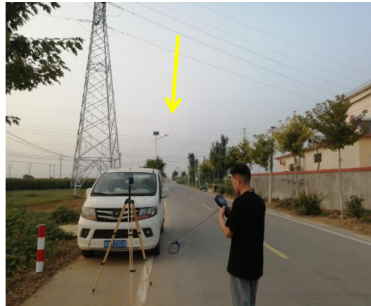
B4:110kV 蒋观线 14#塔~15#杆塔导线衰减
